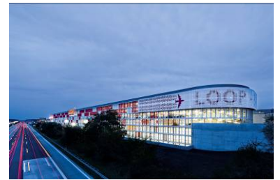
Parking Garage, View A 5
